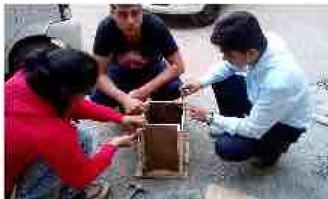
Fig. 18 Assembling of column block formwork
