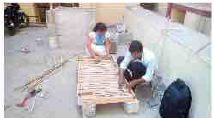
Fig.20 Slab formwork
