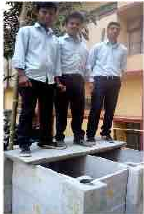
Fig. 24 First testing of slab
