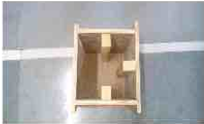
Fig. 17 Groove formwork
